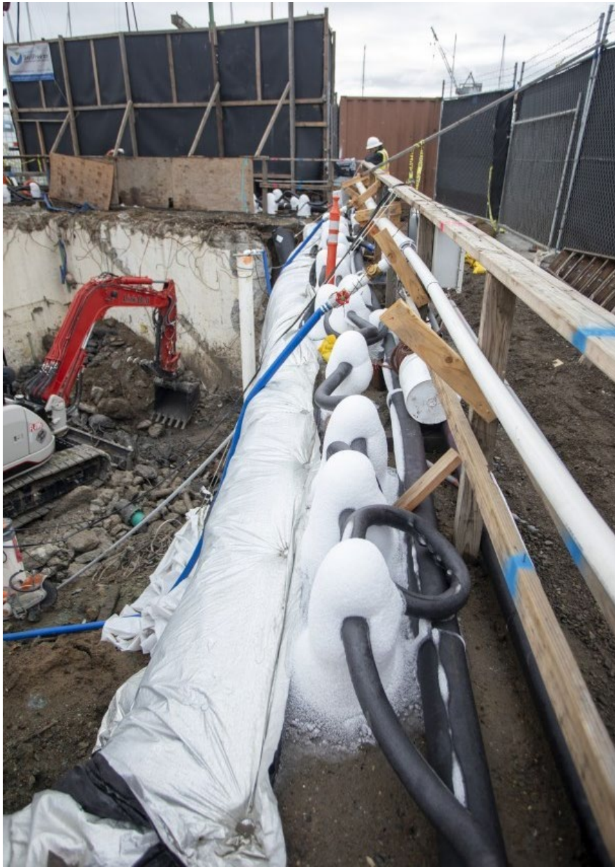
Soil freeze pipes line the outer rim of the excavation site.
